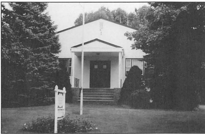
Above, Allendale Municipal Building (in the converted old schoolhouse) on Franklin Turnpike in September 1974. Today this building houses the Allendale Police Headquarters.
