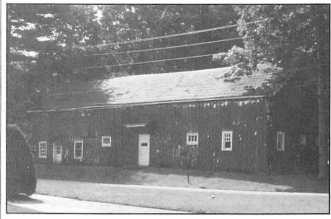
Below, the former Mallinson's Carriage and Wheelwright shop, on what are today the grounds of the Guardian Angel Roman Catholic Church, August 1994.
