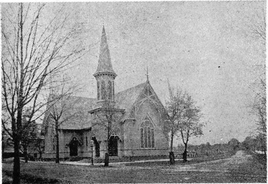
Old Original Archer Memorial Methodist Church
