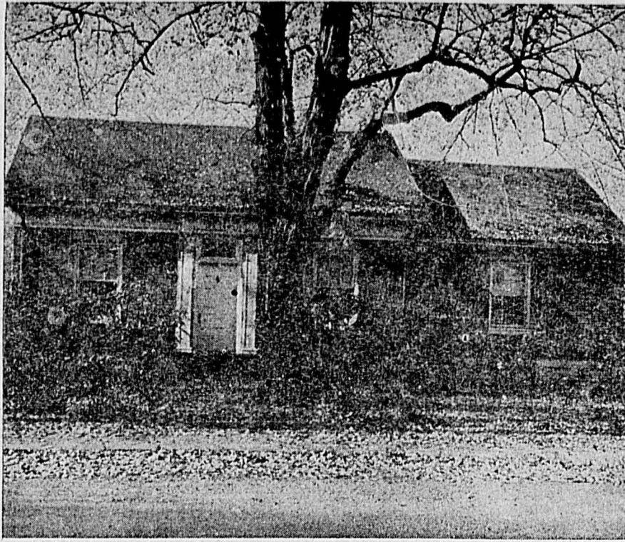
All the trim of the local Library has been painted by the local Lions Club under the chairmanship of Martin Husing. The service organization supplied the materials and labor at their own expense.
