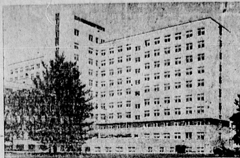
The nine-story 363-bed building at Bergen Pines County Hospital (above) was officially dedicated by the Board of Freeholders, June 7. It is designed for the care of the medically indigent, particularly those suffering from long-term illness. The ninth floor is devoted to the care of short-term mental cases.
