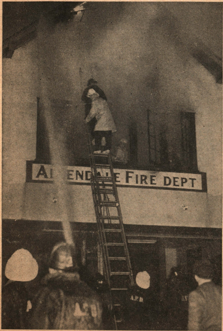
MEMBERS OF the Allendale Fire Department battle a blaze in their own baliwick Thursday as they work to bring under control the early evening fire that destroyed the second floor of the borough's firehouse. The ceiling and furniture in the second-floor meeting room were destroyed and the beams and walls badly charred.
