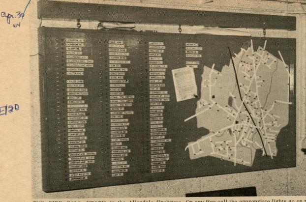
THE FIRE CALL BOARD in the Allendale firehouse. On any fire call the appropriate lights go on to show on what street the fire is located and where that street is located on the borough map at the right.
