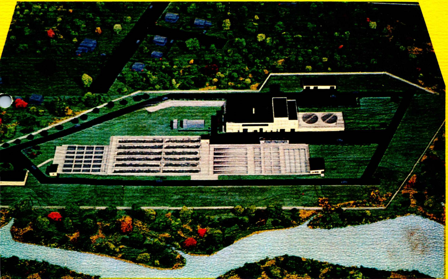
N.W.B.C.S.A. TREATMENT PLANT, Waldwick, N.J.
