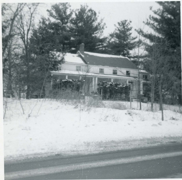
Garrison-Berdan House, Memorial Drive Photographs taken January, 1970.
