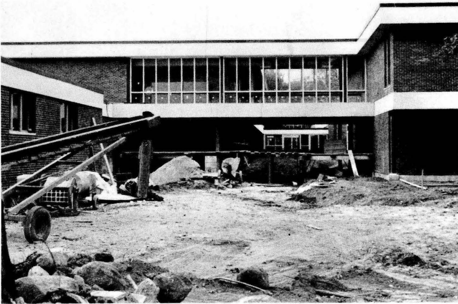
Building addition nears completion.
