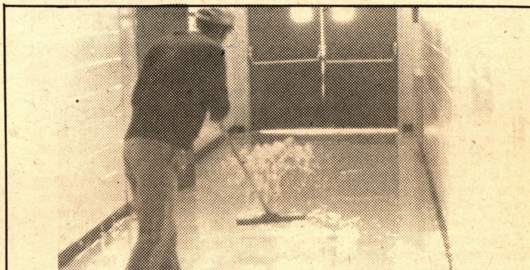
TWO WEEKS AGO, PIPES BURST IN THE PHYSICAL EDUCATION WING AND WATER RAPIDLY FILLED THE CARPETTED WEIGHT ROOM. SOME EQUIPMENT SUFFERED DAMAGE BUT THE MAJORITY OF THE WEIGHTS WERE SAVED. ABOVE, A CUSTODIAN MOPPS UP WATER THAT LEAKED INTO THE GYM CORRIDOR. LATER, A PLUMBING CONTRACTOR WAS HIRED TO EVALUATE AND ADJUST THE MISHAP.
