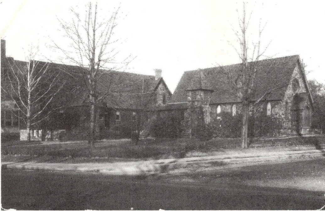
Remodelled and enlarged Chapel building, resituated and attached to Parish House. c. 1907-1910.
