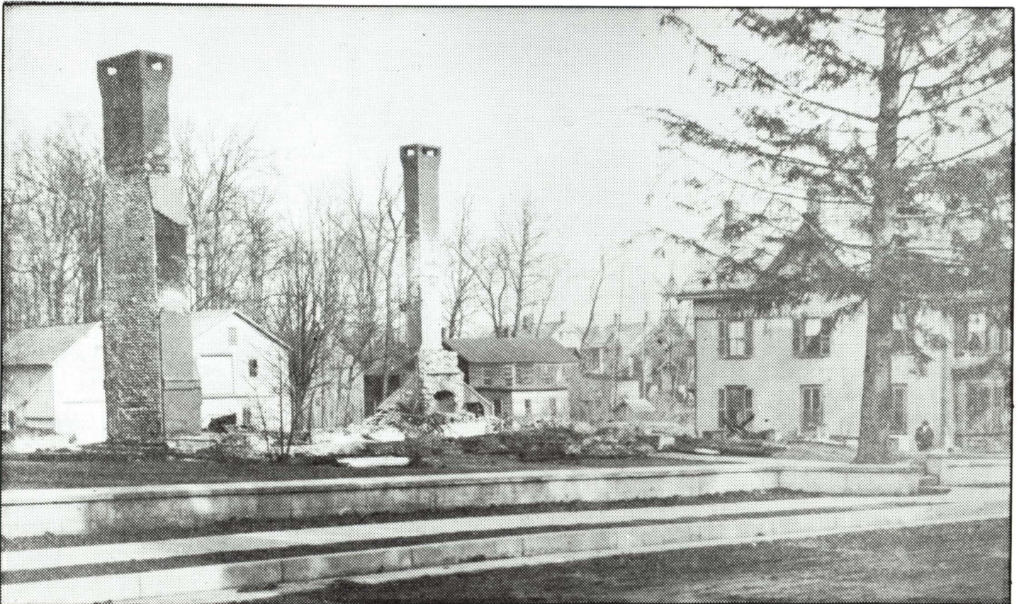
The remains of the mansion of Assemblyman George Cook, 1913. Coal stored in the basement caused the house to smolder for weeks after the fire.
