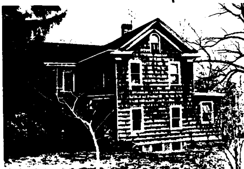
↙ 0201-25 John Christopher House Northeast view, from Park Avenue. Neg. file # 198336-21
