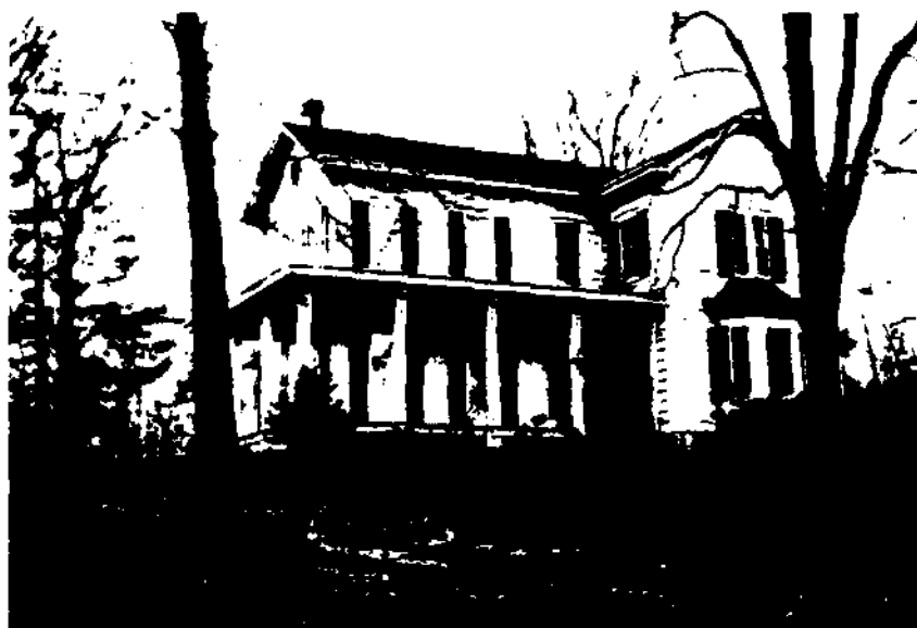
0201-18 Reading House. 509 Franklin Turnpike Neg. file # 198226-22
