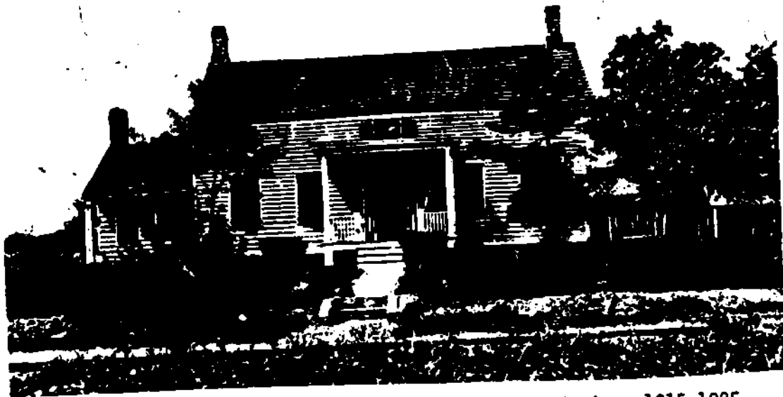
0201-31. Storms-Critchley House, photographed circa 1915-1925. Note the roof height and the altered facade porch (in Colonial Revival style). Photo courtesy of J. Troast, 1985.
