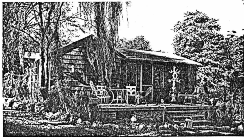
Tax Appraisal Photo, Reconverted Pump House (c. 1947)
