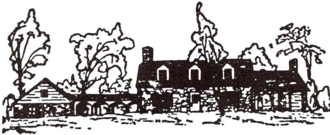
MUNICIPAL BUILDING COMPLETED IN 1981-82
