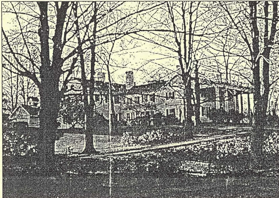
475 Franklin Turnpike, photo taken 1987
