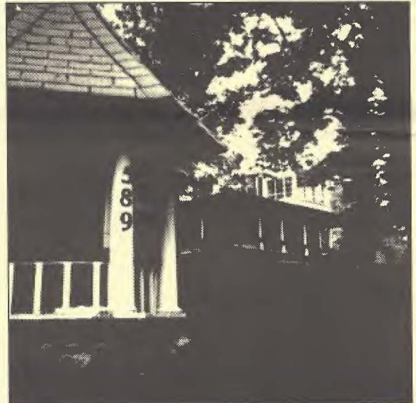
The Van Houten House, 589 Franklin Turnpike. Photo taken June 1987.
