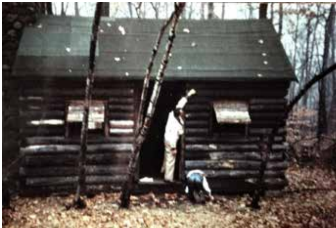
The Cody Log Cabin being repaired by Troop 59 in the 1950's. A fire destroyed the cabin but the chimney still stands today.
